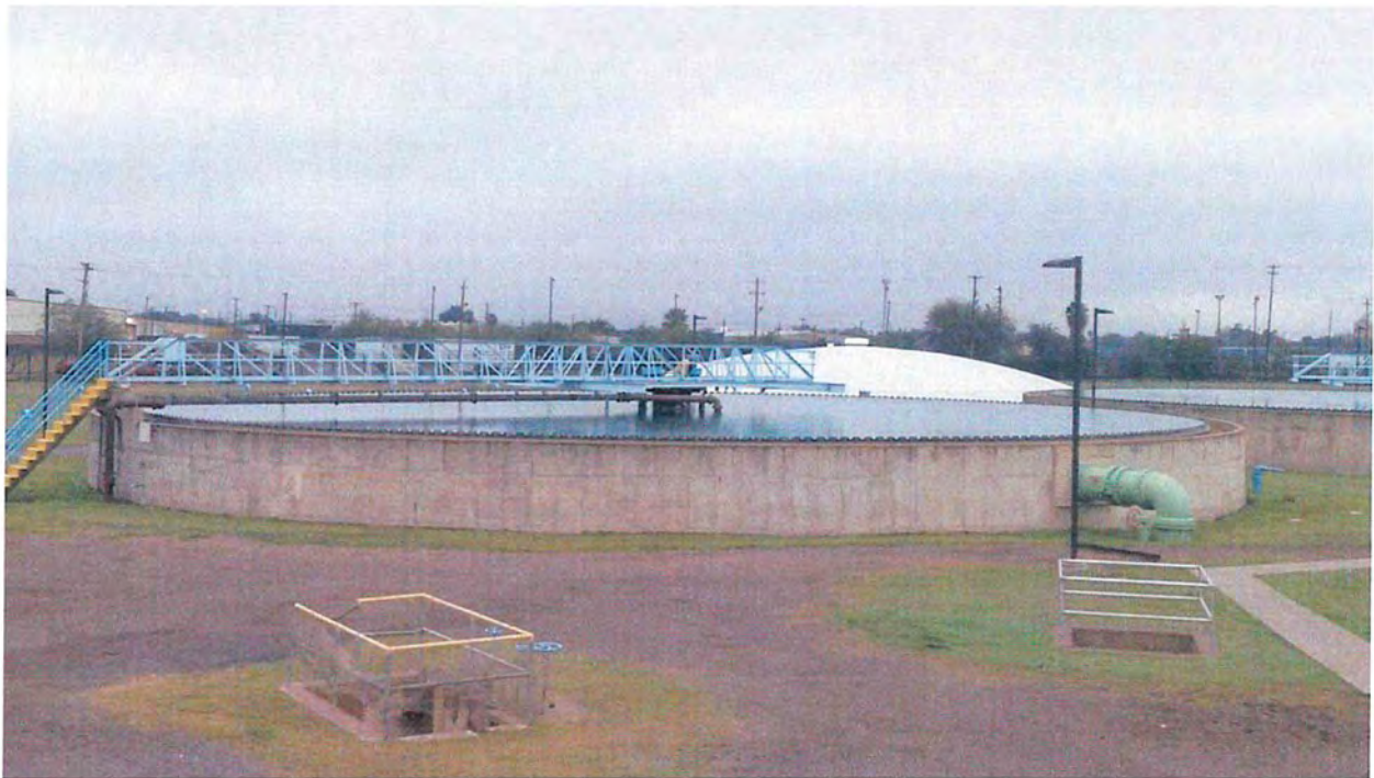
2014-12-19 (14) – North sludge thickener. In service.
