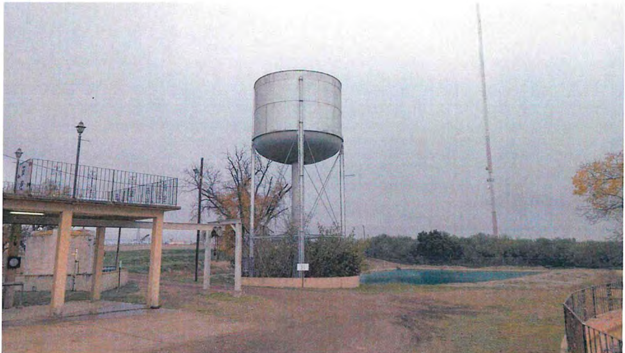
2014-12-19 (10) – Lower plant backwash tank. Not in service.
