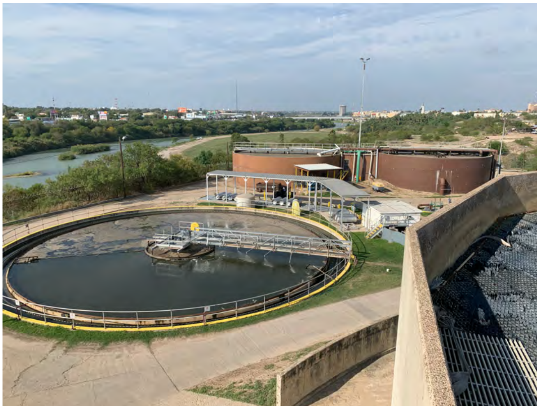
FIGURE 1: TWO RE-AEREATION BASINS, SECONDARY CLARIFIERS, CHLORINATION SYSTEM
