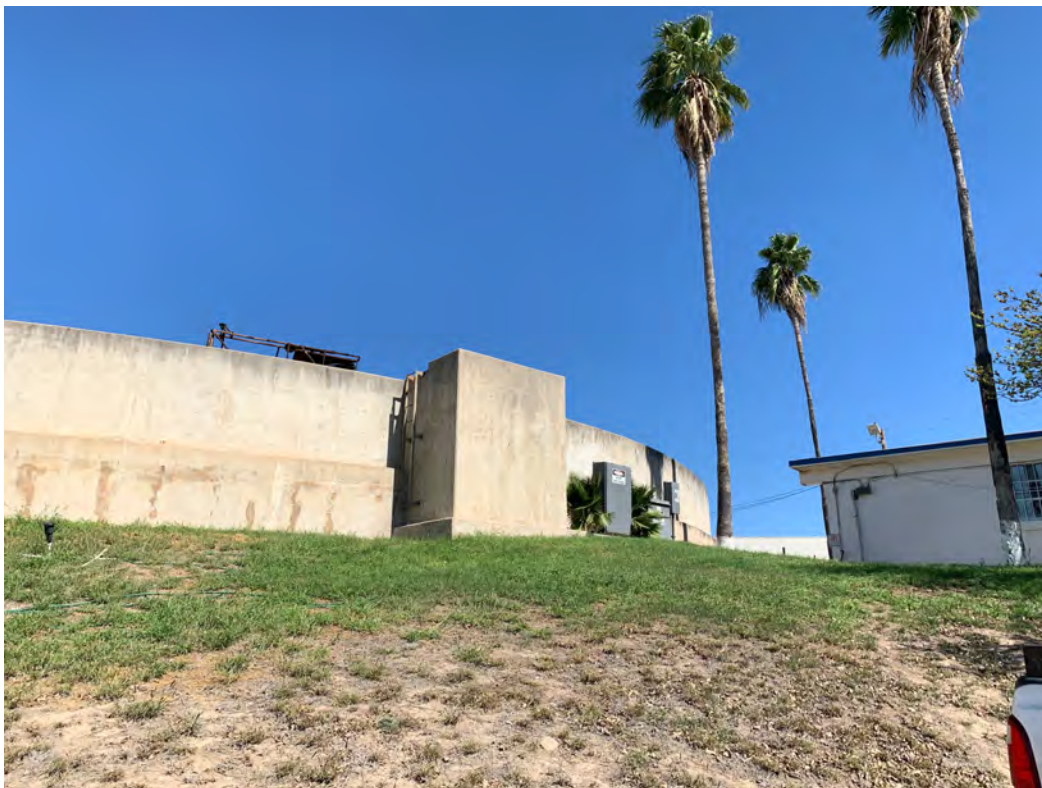
FIGURE 3: ABANDONED TRICKLING FILTER AND ZCWWTF OFFICE BUILDING
