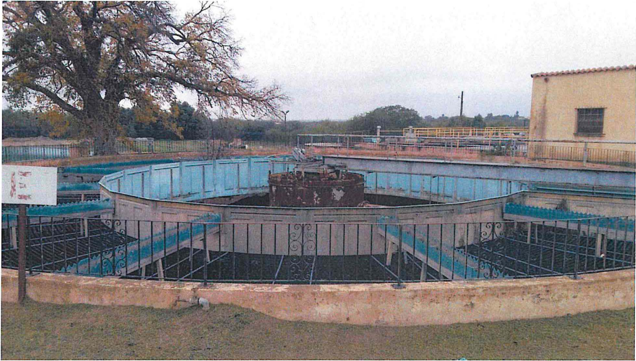
2014-12-19 (03) - One of two sedimentation basins in the lower plant. No longer in service. Nothing in the lower plant is in service any longer.
