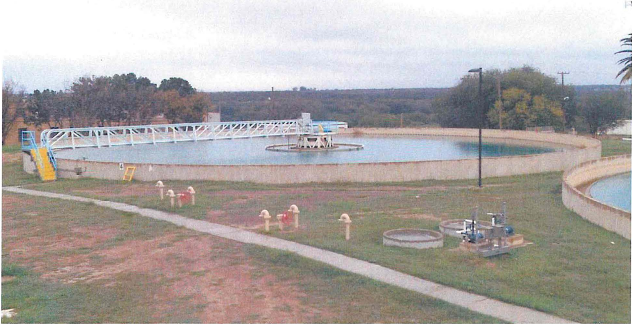
2014-12-19 (11) – Clarifier 4. In service.
