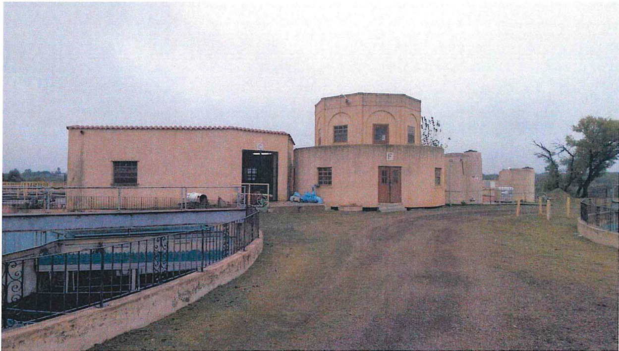
2014-12-19 (04) – Maintenance storage and chemical injection in lower plant. Not functional. Used as storage.
