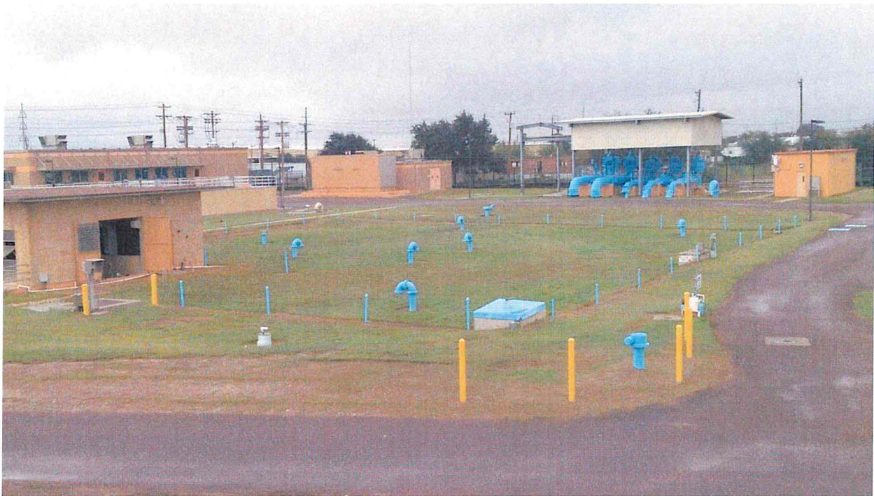
2014-12-19 (18) – Clearwell 1 (underground). In service.
