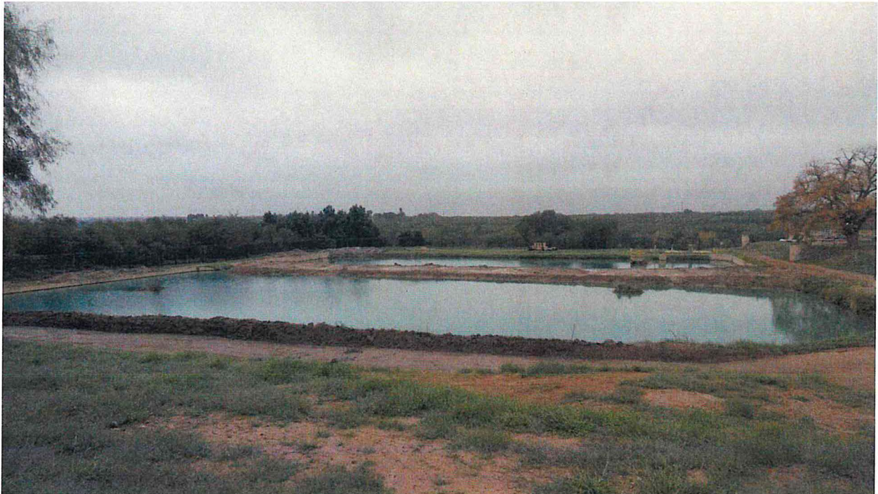
2014-12-19 (02) - Sludge Settling Lagoons.
