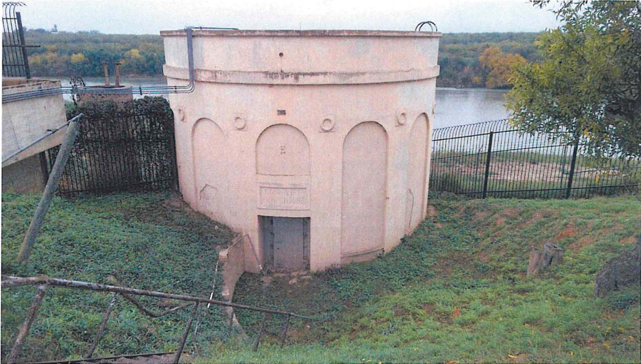
2014-12-19 (07) – Original lower plant pump house. No longer in service.
