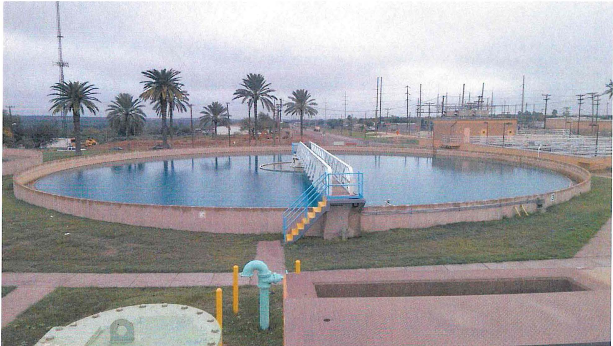
2014-12-19 (12) – Clarifier 3. In service.
