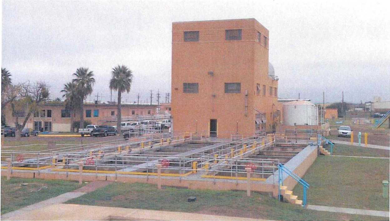
2014-12-19 (13) – Flocculators (from left) 3A, 3B, 4A, 4B, all in service. Old chemical injection building, no longer functional, used for storage.
