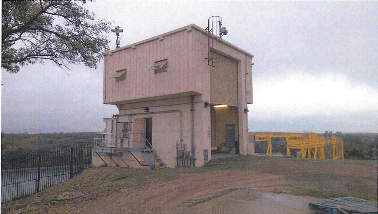
2014-12-19 (09) – Lower plant pump house. In service.
