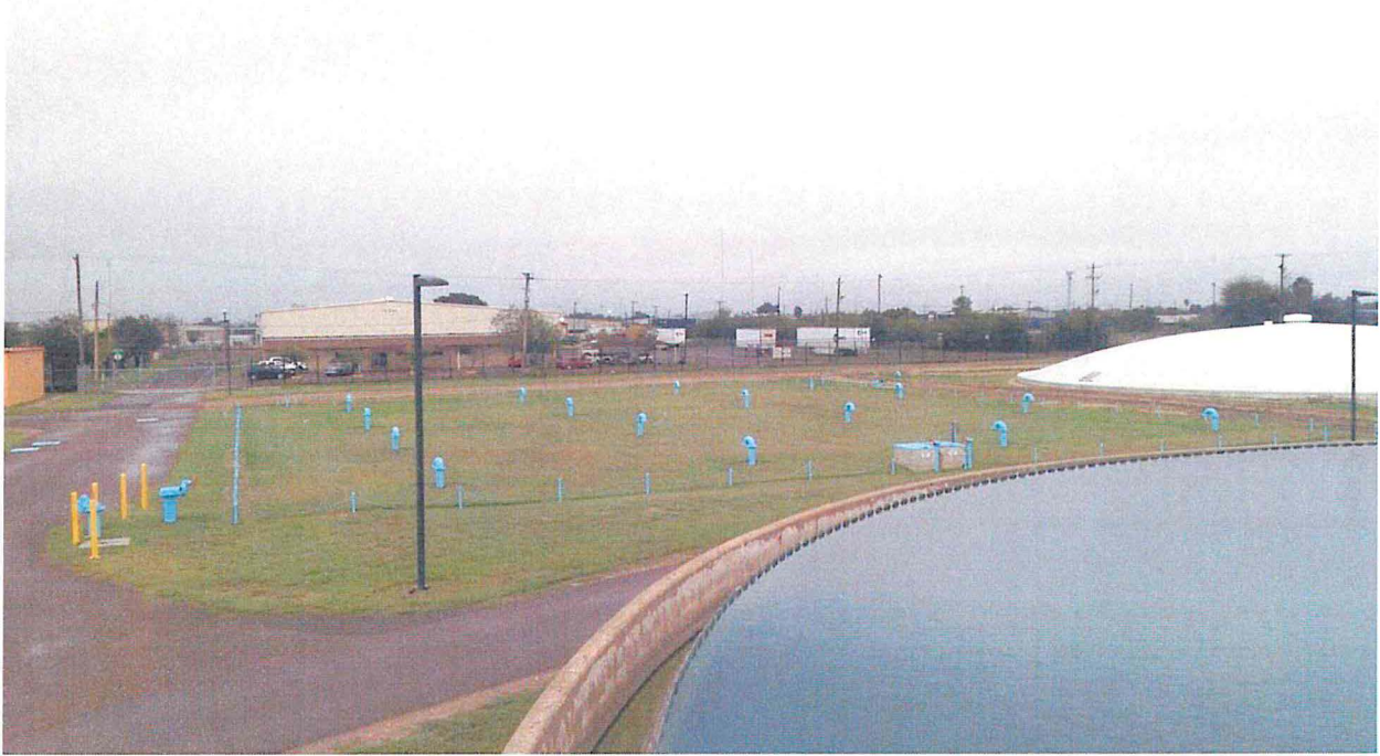
2014-12-19 (19) – Clearwell 2 (underground). In service.
