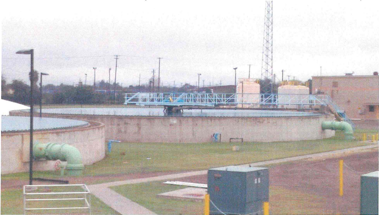
2014-12-19 (15) – South sludge thickener. In service.
