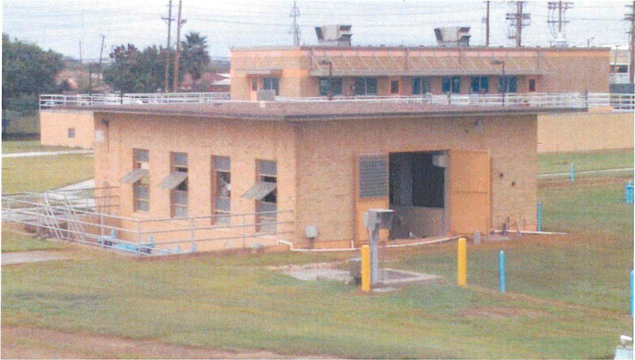
2014-12-19 (17) – West High Service Pump House. In service.
