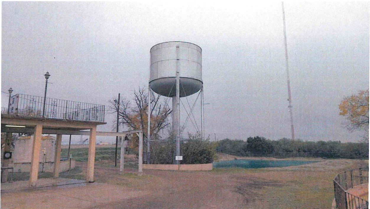
2014-12-19 (10) – Lower plant backwash tank. Not in service.
