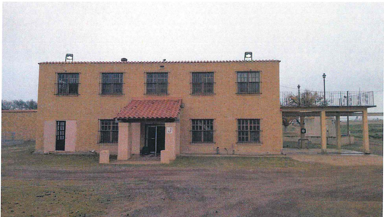
2014-12-19 (06) – Lower plant administration and filter building. No longer in service. Used for storage.
