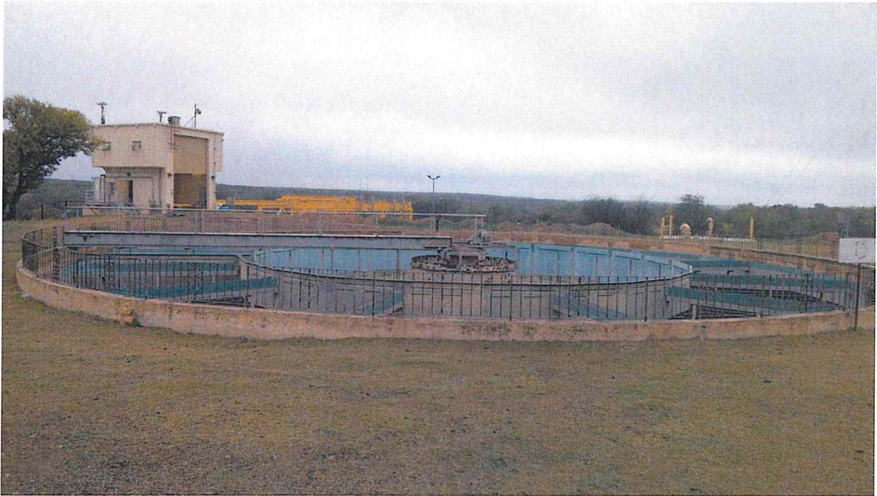
2014-12-19 (05) - One of two sedimentation basins in the lower plant. No longer in service.
