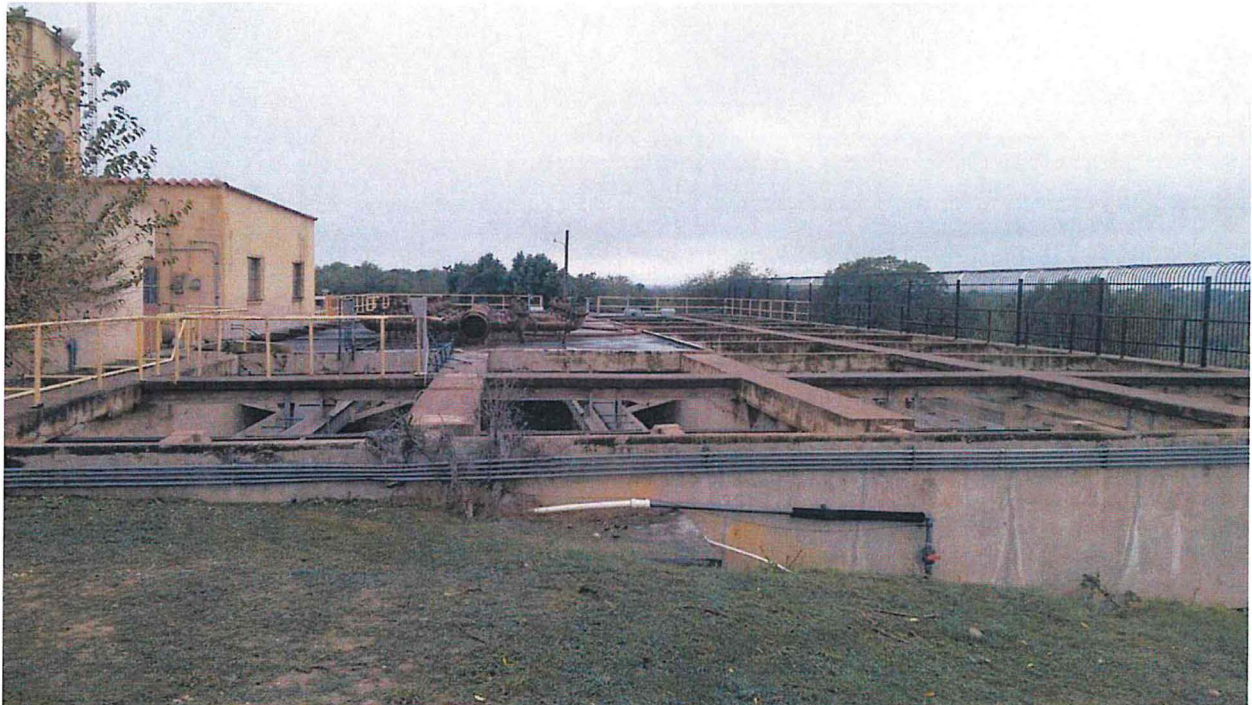
2014-12-19 (08) – Lower plant aerator and flocculators. No longer in service.
