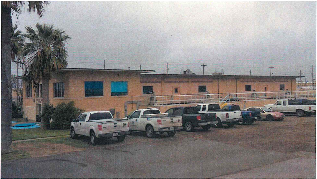
2014-12-19 (01) - Filter Building 1. The front half was erected c1954, as were most of the items in the following pictures. Only the first four filters were built then. The last four filters were added c1975. The 1954 part is everything to the left of the last two large windows on the right.
